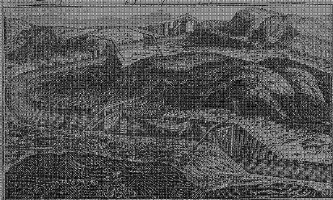
Fig. 2. Section of a LOCK.
